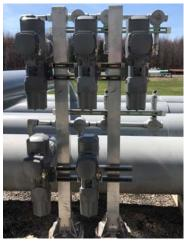
One of the largest Natural Gas Transmission Utilities in North America awarded R.M. Headlee Co., Inc. with two orders for AUMA electric valve actuators. These explosion proof actuators are installed at a transmission compressor station on ANSI Class 600 suction, discharge and by-pass API-6D trunnion ball valves and plug valves.
