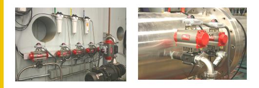
When our client needed new equipment assimilate space conditions thev to turned to the expertise of R.M. Headlee Valves & Controls and the proven performance of A-T ball valves. The requirement was to test a multitude of gases under full vacuum and extremely high flows in an aerospace wind tunnel utilizing automated ball valves. A-T was able to provide "leak free" valves by specially machining the seat configuration and reengineering the packing design. By
