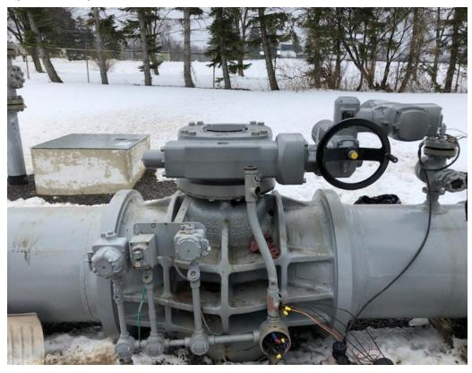
there were no records or torque information available. Therefore, all valve dimensions were measured in the field to assure correct machining of adaptation and mounting plate, which aided in an efficient installation. This particular valve is on the primary discharge pipeline for 900-psig natural gas from the compressor station.
